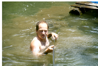
River bed maintenance in Costa Rica
